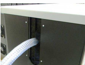
Pipe and cable are going through a polypropylene brush
